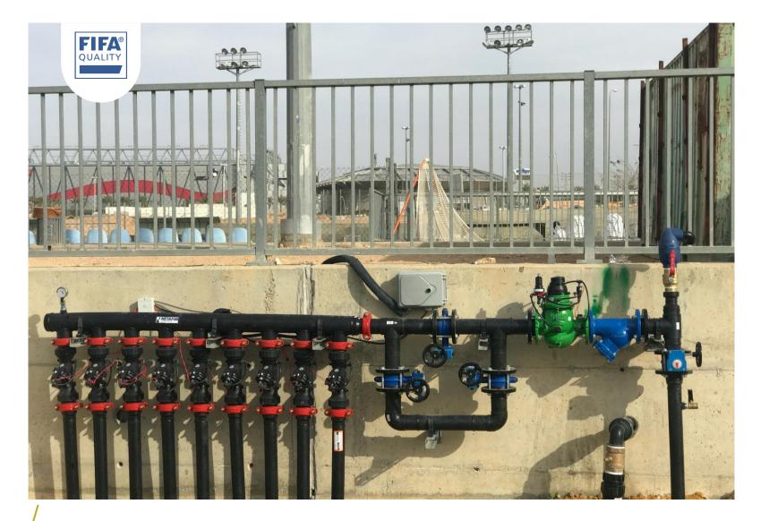
Manifold for the training group of the alumni group includes pressure pump preparation, from the operating system through a local controller with remote control preparation.
