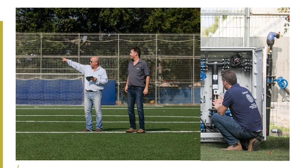
After the assembly is complete, we perform an initial system operation - in this session we perform a system inspection in terms of several parameters: program / assembly compatibility, accessory connection testing, system dryness (no fluidity), anchoring and fixing the system, etc.
