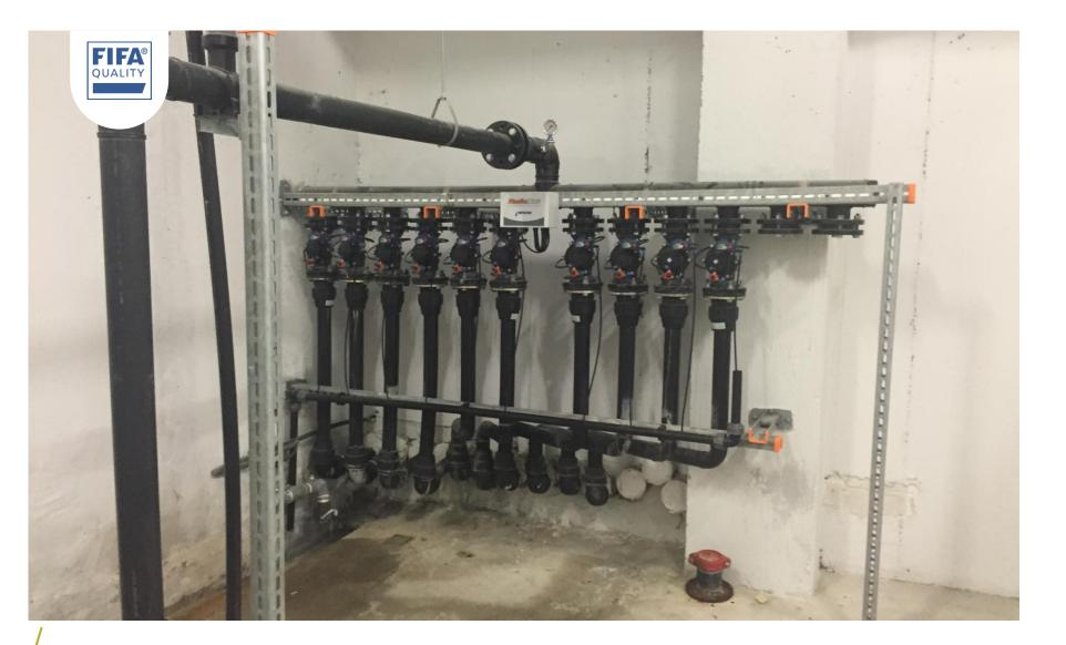
Water chamber with two different water sources - reservoir water and water sources, a pressure boost system with a groundfloor pump CR64 and an automatic filter include dripping valves and main control valves for the system
